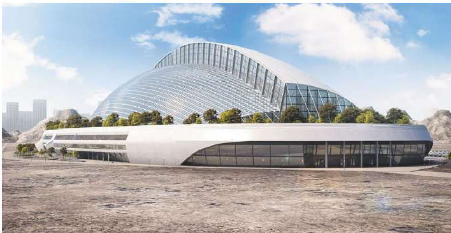
Figure 16 – Rendering of ECH-Earth (option) with a structural solution in the form of torus fragment with a longitudinal section and a raised part of roofin
