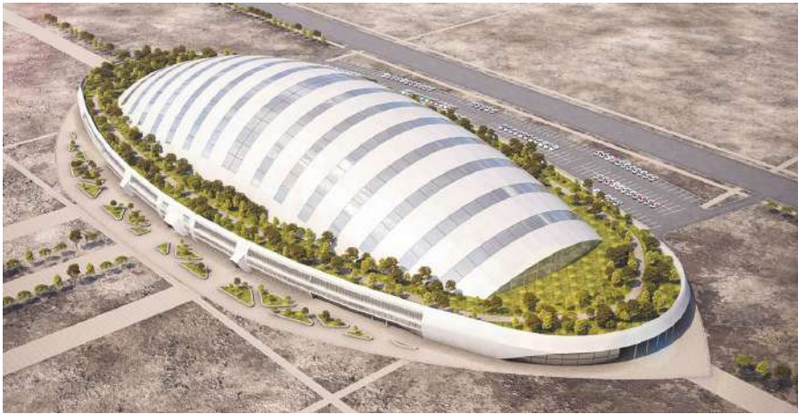
Figure 15 – Rendering of ECH-Earth (option) with a structural solution in the form of torus fragment (height – 30 m)
