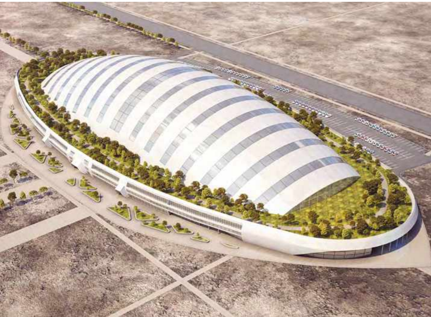
Figure 15 – Rendering of the ECH-Earth (option) with a structural solution in the form of a torus fragment (height – 30 m)
