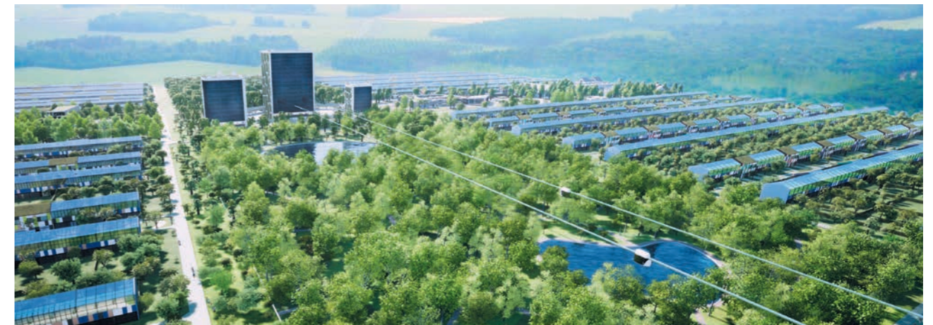
Figure 8 – View at the residential cluster recreational area (variant)
