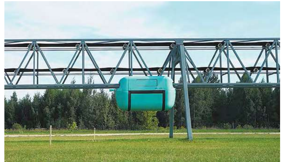
Testing of unitruck. EcoTechnoPark, Maryina Gorka, 2018
