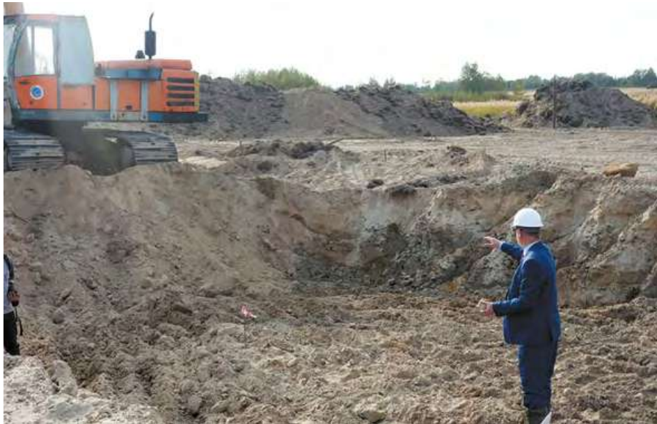
Excavation for the anchor support in EcoTechnoPark. Maryina Gorka, August 2015
