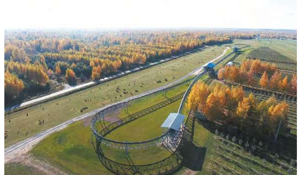
SkyWay cargo complex, the overpass of which has two structures: a conveyor belt (unitrans) and cargo modules (unitruck). EcoTechnoPark, Maryina Gorka, 2018.
