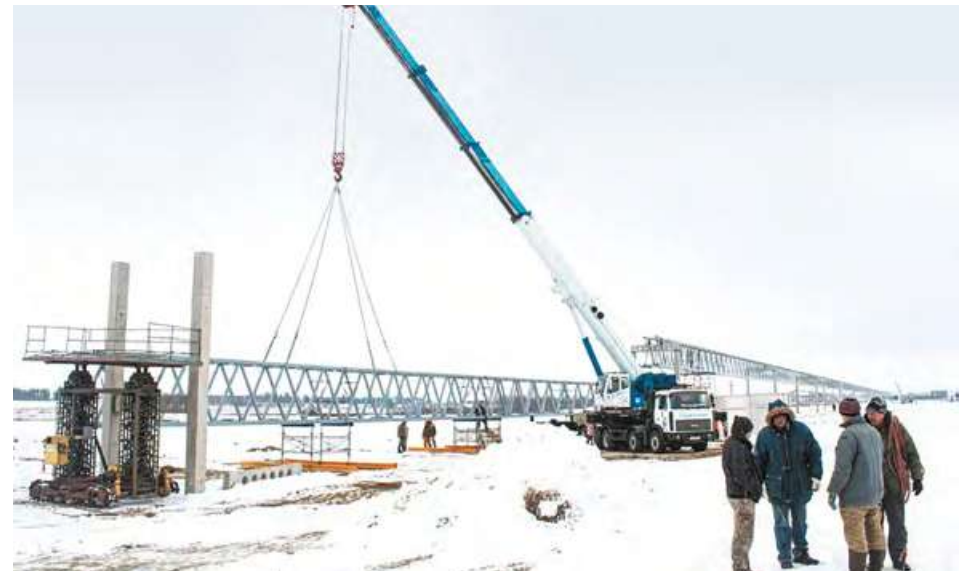
Installation of the trusses of the urban track structure. EcoTechnoPark, Maryina Gorka, February 2017
